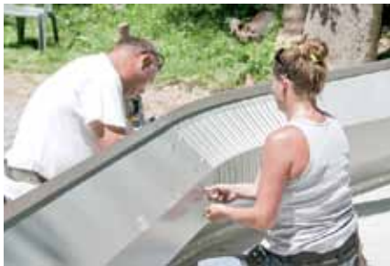
Bolt arches together on the ground
