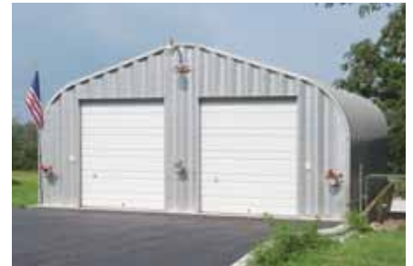
Install doors and endwalls
