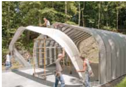
Raise the arches into place
